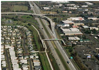
Interstate 5/Beltline/Gateway Construction
