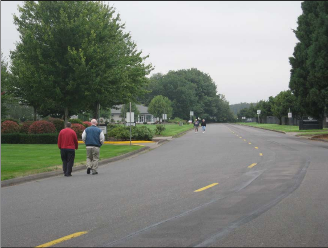
Pedestrians on roadway along Coburg Industrial Way
