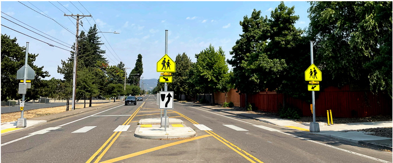
A pedestrian crossing with Rectangular Rapid Flashing Beacons.
