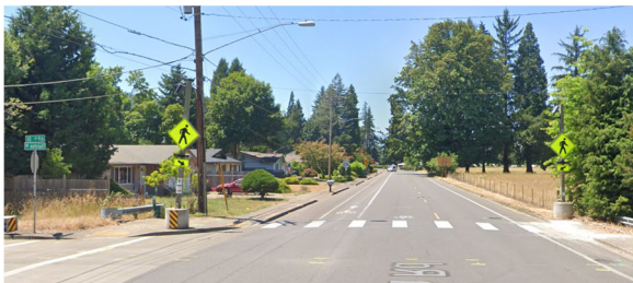
Temporary RRFB at Thurston Rd at 69 th St that will be replaced by a permanent crossing with this project
