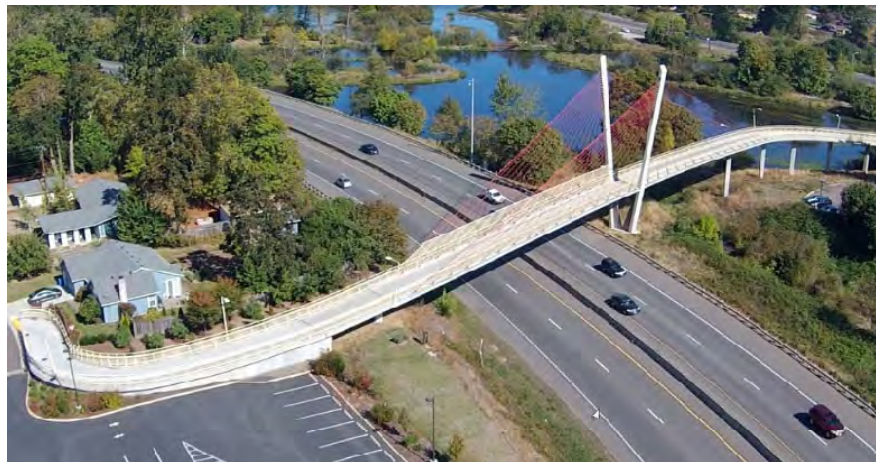
Photo of Delta Ponds bicycle and pedestrian bridge in Eugene. The River Road-Santa Clara pedestrian and bicycle bridge would provide a similar connection over the Randy Papé Beltline, though will likely be a different style of bridge.
