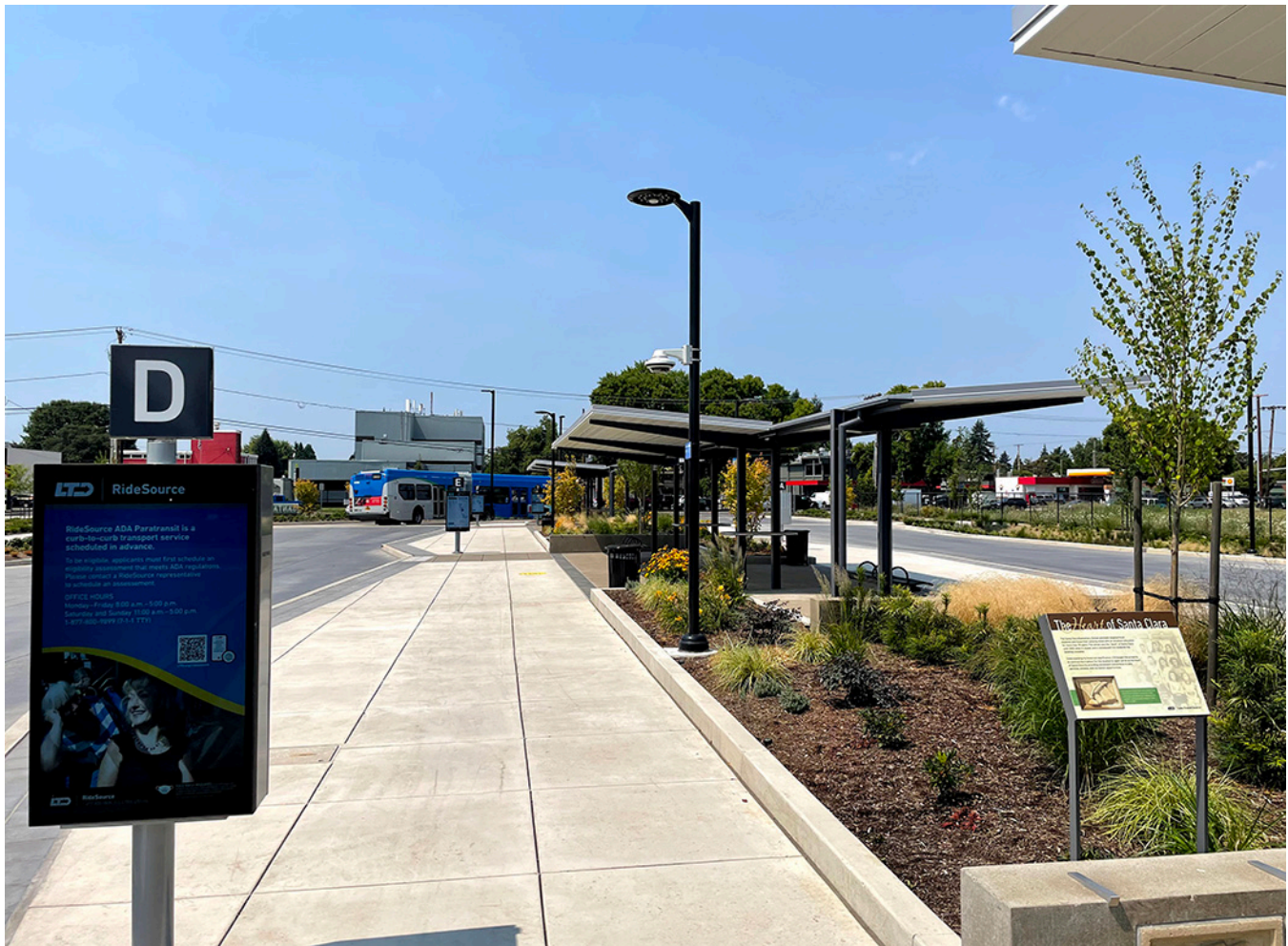
A bus departs from the Santa Clara transit facility.
