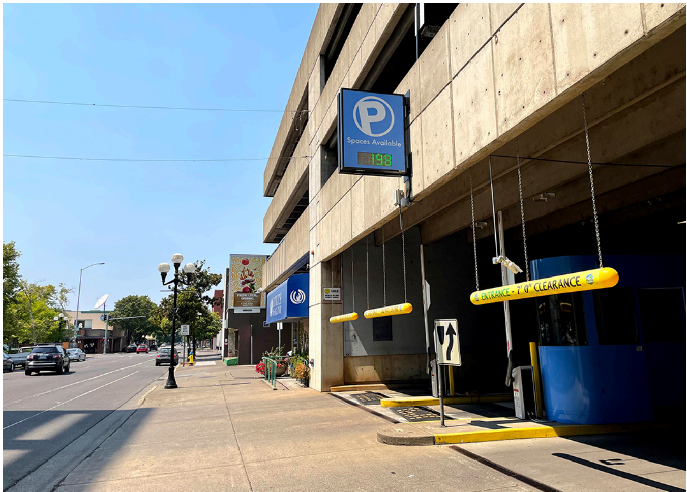
A parking garage in downtown Eugene.
