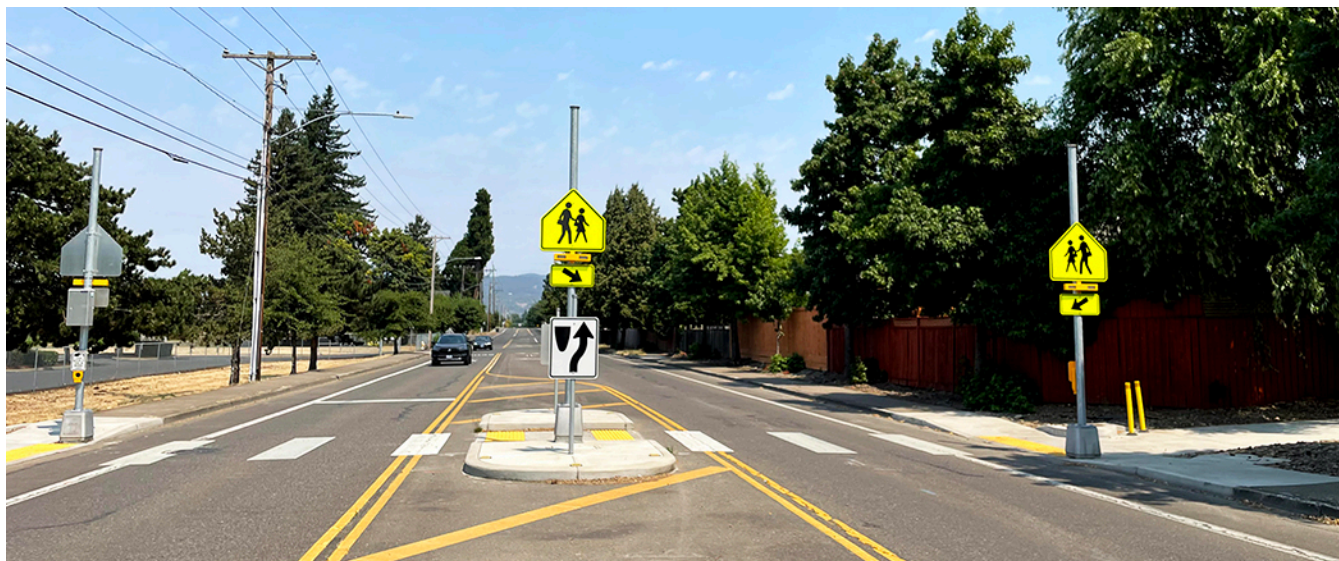
A pedestrian crossing with Rectangular Rapid Flashing Beacons.
