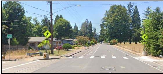
Temporary RRFB at Thurston Rd at 69 th St that will be replaced by a permanent crossing with this project
