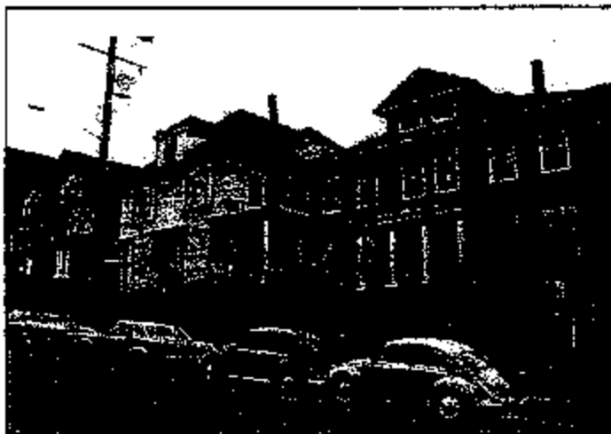
Houses prior to renovation
