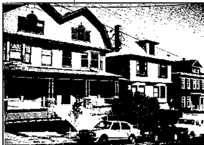
Street view of three houses after renovation
