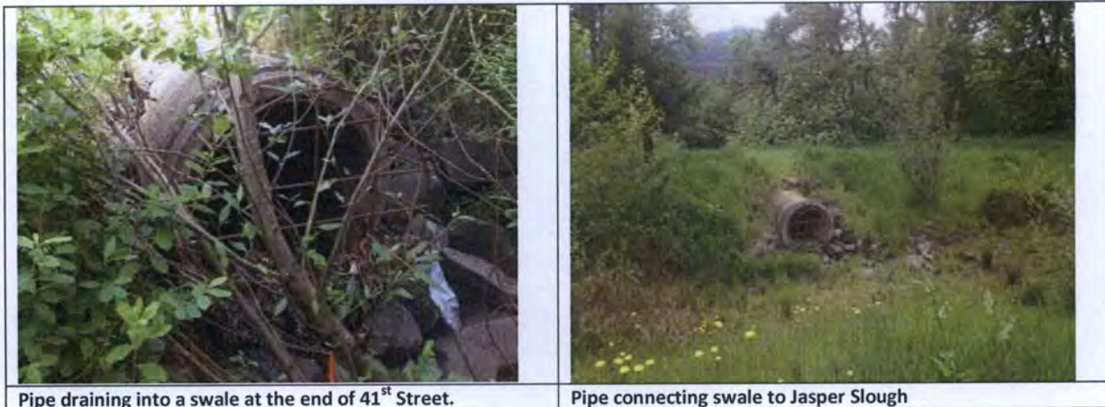
Pipe draining into a swale at the end of 41 st Street.
