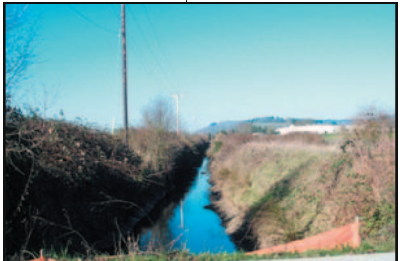
Muddy Creek Irrigation Channel
