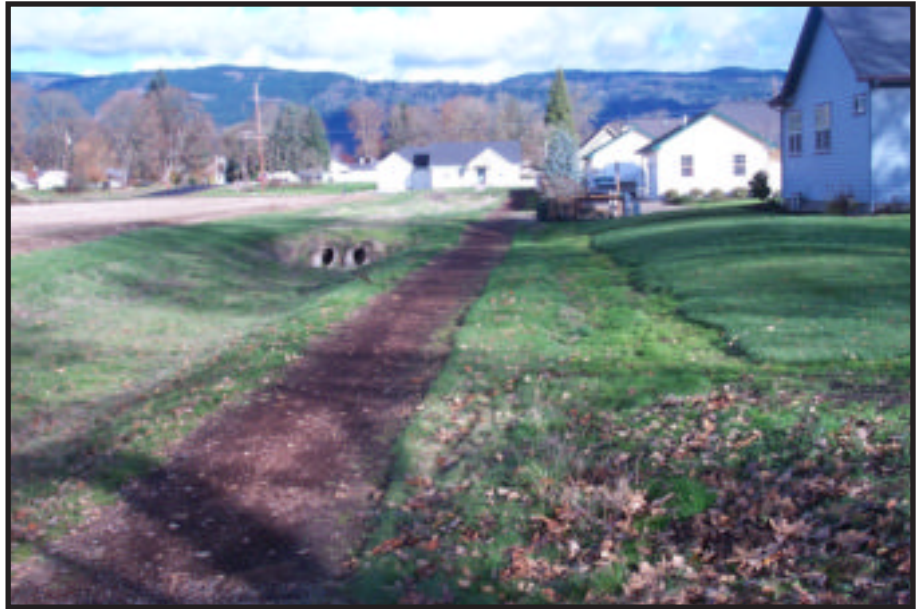
A portion of the path will parallel the City owned Bio-Swale near Bruce Street.
