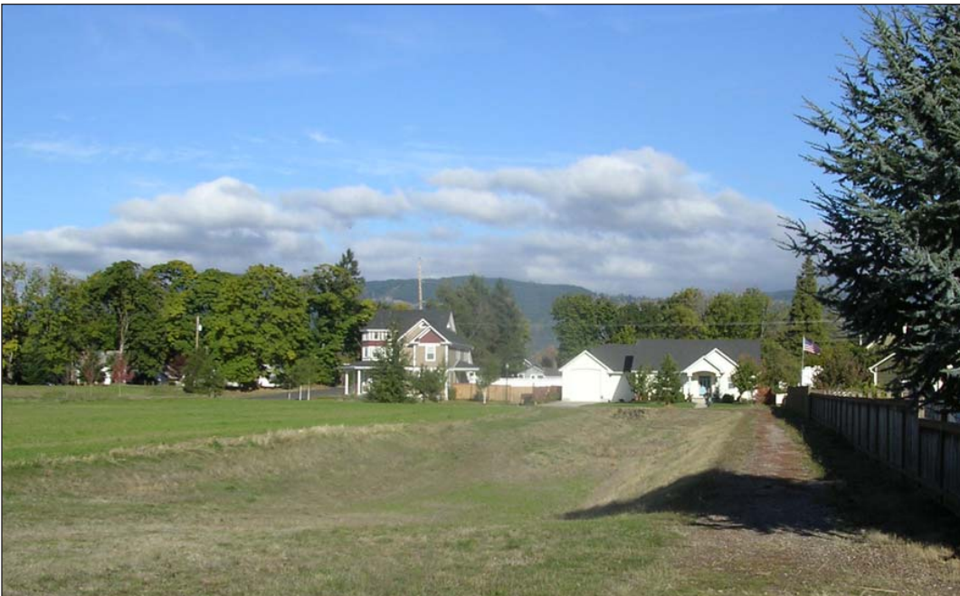
Bioswale near Canterbury Slough in Northwest Coburg — Among the sustainability goals and policies, Coburg aims to encourage infill development, preserve its open space, and protect adjacent agricultural lands.
