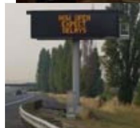
Permanent Dynamic Message Sign
