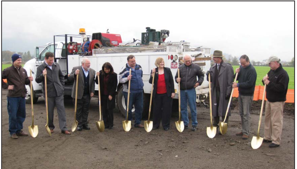
Coburg Wastewater Groundbreaking for Treatment Facility and Collection System (left to right) John Thiel, City Councilor; Nick Batz, representing Congressman DeFazio; Phil Barnhart, State Representative; Juine Chada, representing Senator Wyden; Faye Stewart, Lane County Commissioner; Judy Volta, Mayor; Jerry Behney, Councilor; Jae Pudewell, Council President; John Fox, Councilor; and Don Schuessler, former City Administrator.
